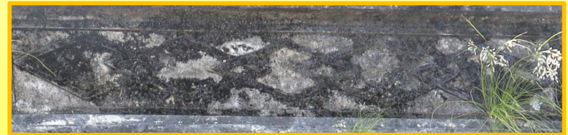
屋頂女兒牆的裝飾構件 Decorative features on roof parapet
